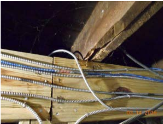
Figure 14: Existing Termite Distress @ Floor Joists
