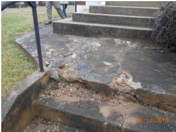
Figure 3: Concrete Pier Settlement
