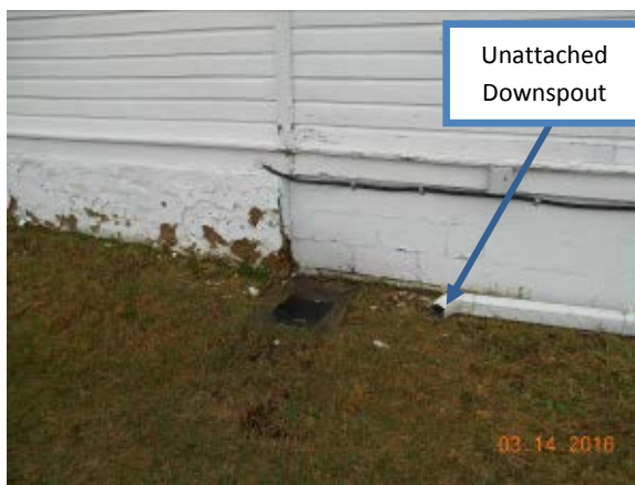
Figure 6: Unattached Downspout.
