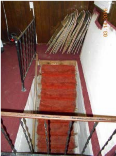
Figure 16: Interior Basement Access Stairs.
