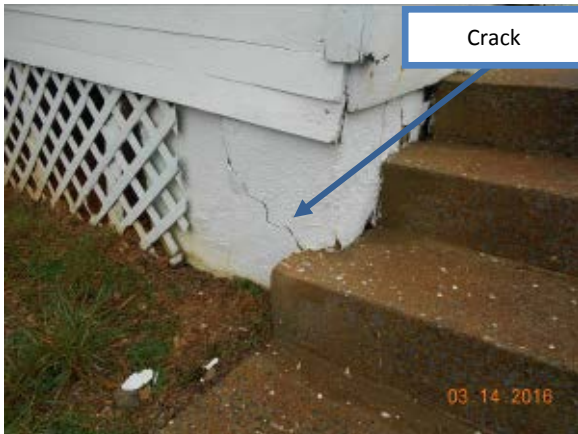
Figure 3: Concrete Pier Settlement
