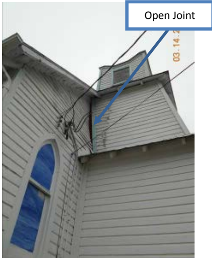
Figure 2: Main Church and Bell Tower Separation.
