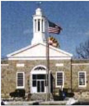
Town of Bel Air's former post office building
