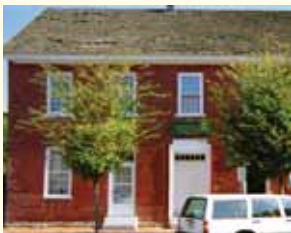
Chester River Hospital Center
