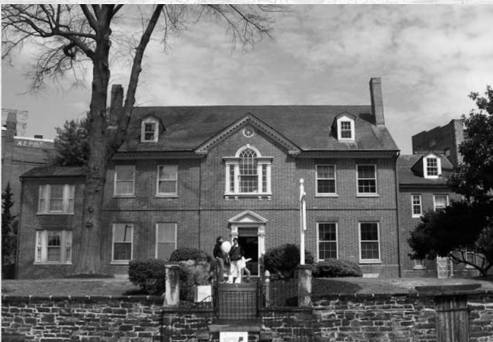
The Old St. Paul's Rectory was restored by PM in the 1980s and serves as its headquarters.
