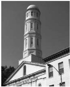
Tower before restoration
