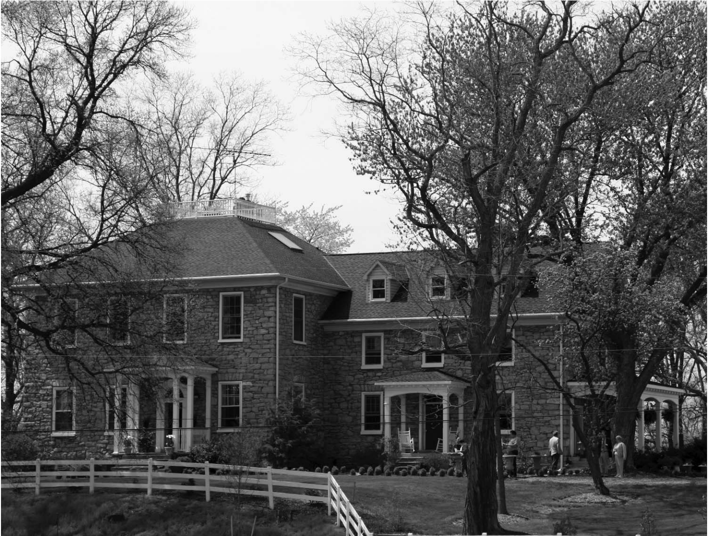
Rockland – located on Sharpsburg Pike in Washington on County
