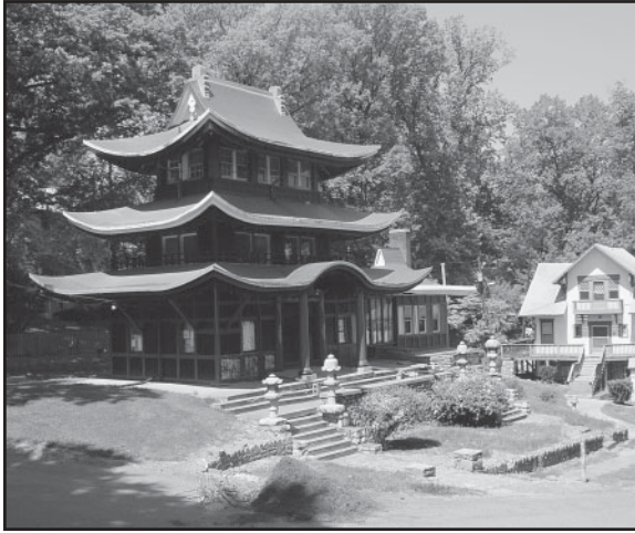
The restoration of the Pagoda is a current project initiated by Save Our Seminary, a local non-profit organization dedicated to protecting the National Park Seminary's historic resources. In the future, SOS hopes to utilize the Pagoda for a visitors center and museum.
