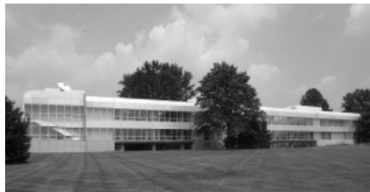
The COMSAT building, designed by Cesar Pelli in 1969, is currently threatened by intense development pressure. Without designation as a Montgomery County Landmark by the County Council, this highly significant structure could be demolished in favor of new construction.
