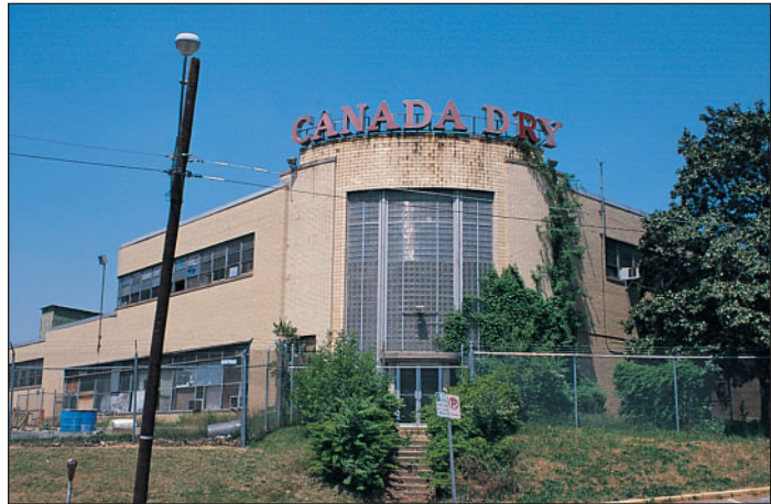
Preservation Maryland joined with local advocates to oppose the demolition of the Canada Dry Bottling Plant in Montgomery County and to seek historic designation for the 1946 structure.
