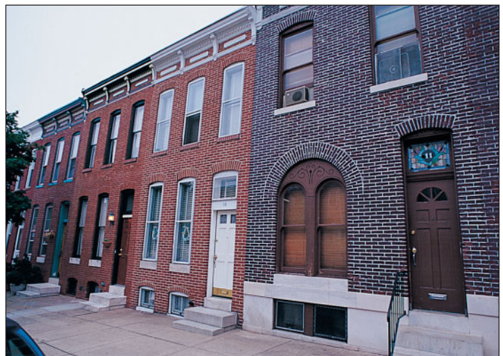
Patterson Park/Highlandtown Historic District is renowned for its distinctive rowhouses that housed a variety of working class immigrant groups in the late 19th and 20th centuries. With 5,208 contributing buildings, the Patterson Park/Highlandtown National Register nomination was the largest assisted by the Historic Communities Investment Fund.
